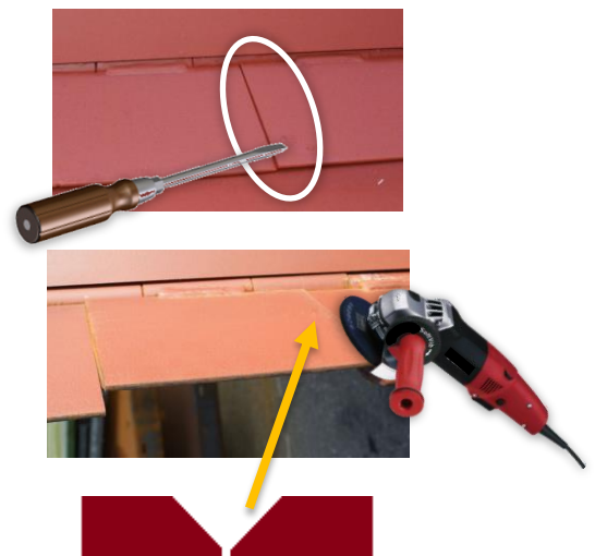
Fig. 95: Checking the scrapers
